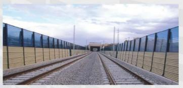
\*Above images serve as examples of noise mitigation measures and are not an indication of a preferred method for use on the California High-Speed Rail project
